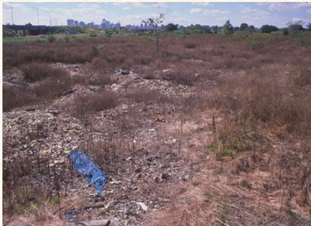
The landfill in 1991. The site was covered with 24" of subsoil and 12" of topsoil. Source: Corbin et al., 2016.
