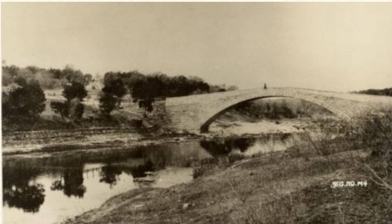
Upper Barton Creek Bridge, late 1800s, shows bank erosion from lack of dense tree cover. Source: Chalberg Collection of Prints and Negatives at the Austin History Center.
