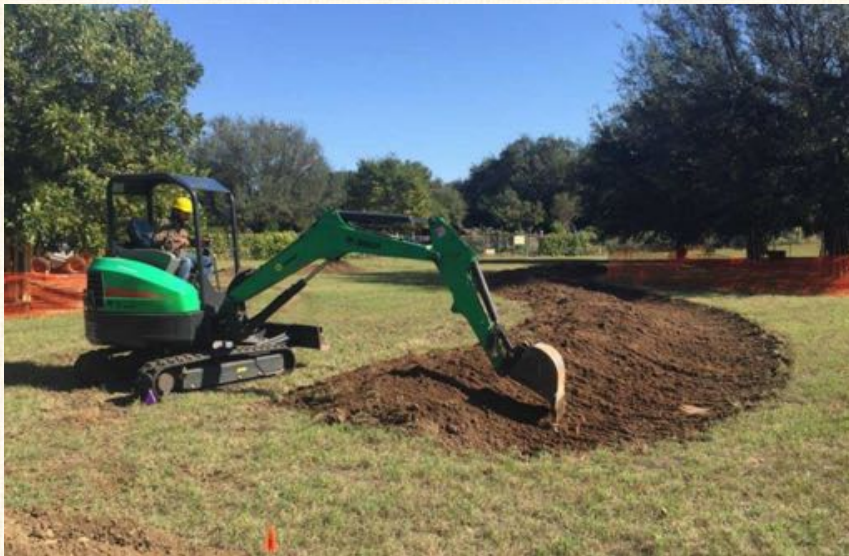
Contour-swales can be added to compacted soils that include shallow caliche. Source: Drought Proof Texas at Austin's Festival Beach Food Forest.
